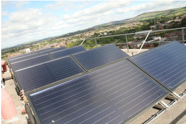
Solar Thermal (hot water)
