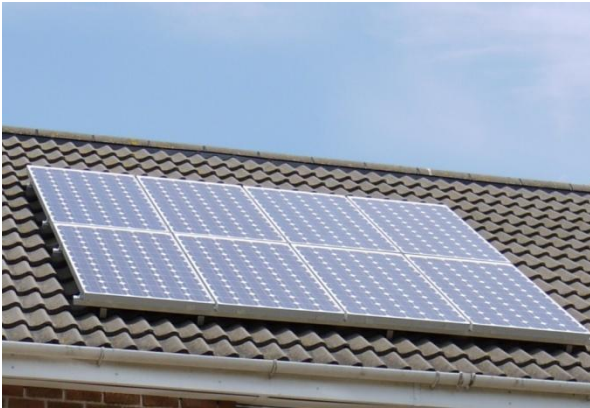
Solar Photovoltaic (PV)
