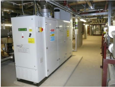
Figure 7: Energ100kWth, 70kWe gas-fired CHP plant, installed at Highbury Stadium redevelopment, London.
