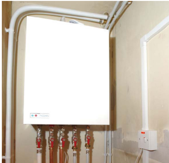
Figure 3: A heat exchanger inside one of the flats connected to the Aberdeen district heating network (Source: Aberdeen City Council: a case study of community heating CE65, Energy Saving Trust, 2003)
